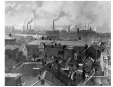
The Krupp works in Essen , 1890
